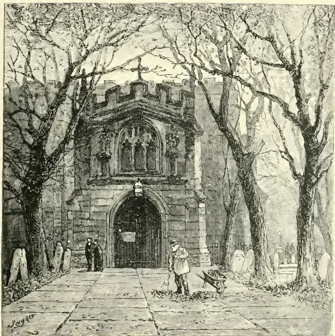
PORCH, STRATFORD CHURCH
